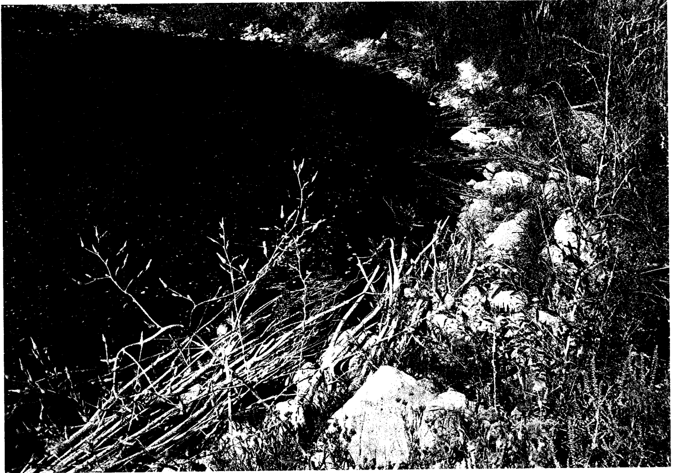
Restored streambank on Squaw Creek.
