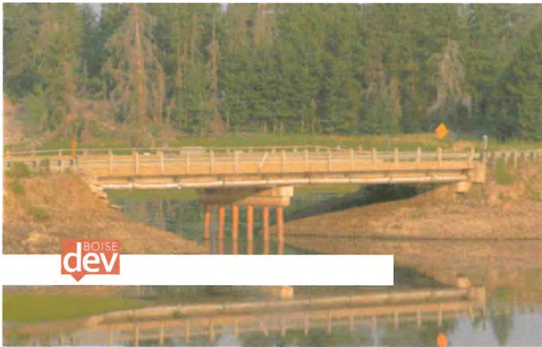
The S-bridge. Photo courtesy of Jeff McFadden.
