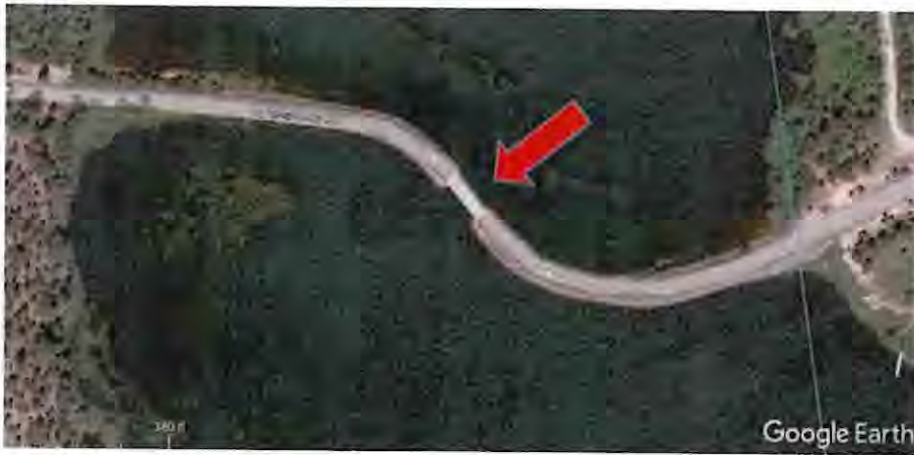
Figure 3; Roseberry Road S-Bridge, an aging infrastructure and scene of numerous accidents.
