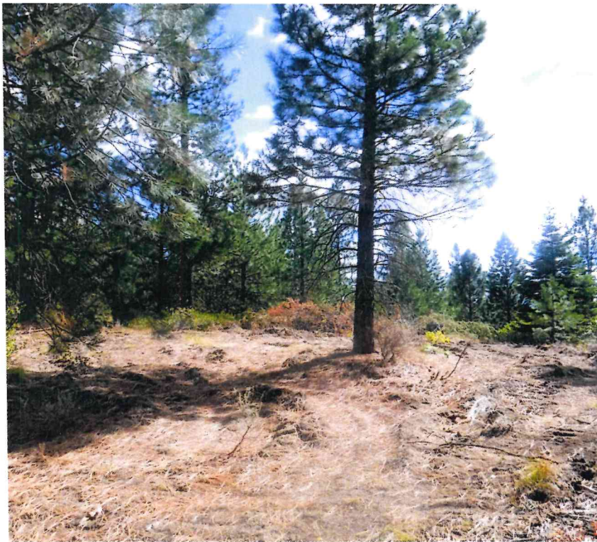
Figure 6: Clearing and masticating for a future building site.
