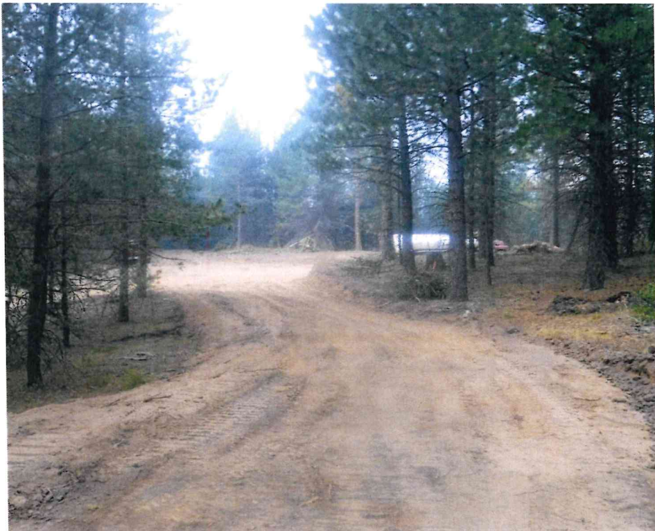
Figure 3: Current driveway that has been constructed.
