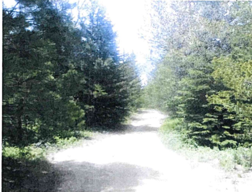
Portion of Laurins Lane that needs reconstruction to meet county standards and a shaded fuel break installed on both sides of the road.
