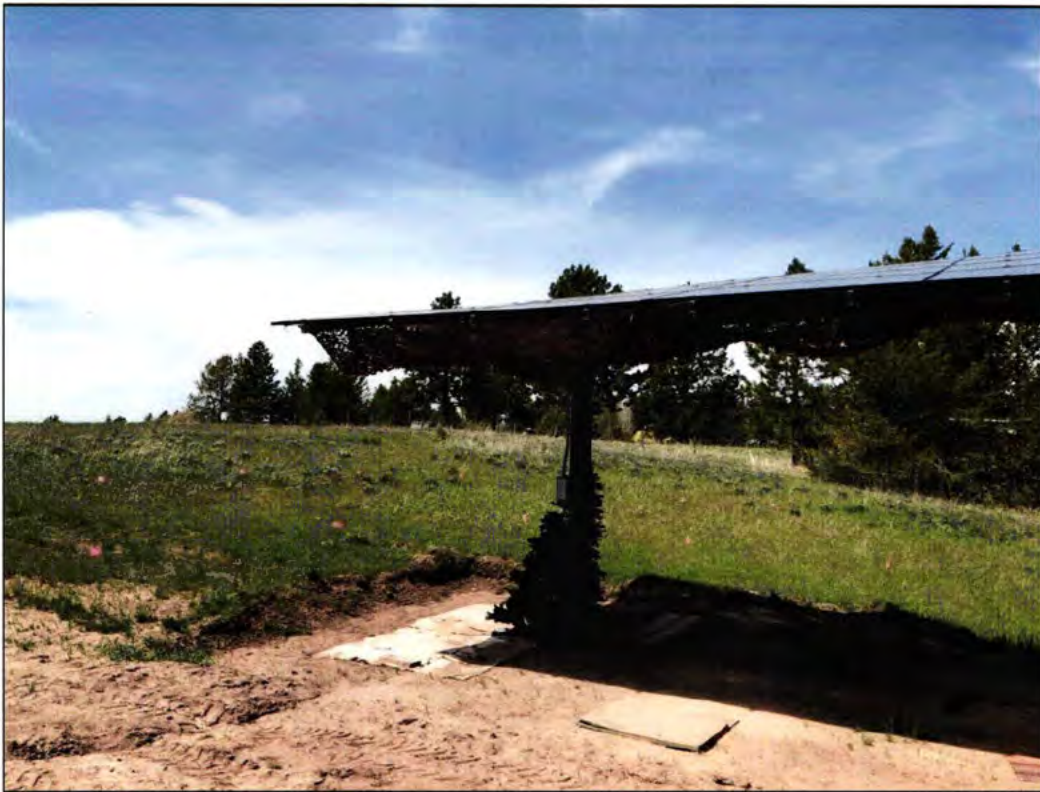
Photo 10. View looking north/northwest at solar array directly north of garage. The camouflage netting was not intended to be a permanent solution for screening. Photo: Mark McClellen 5/10/2026
