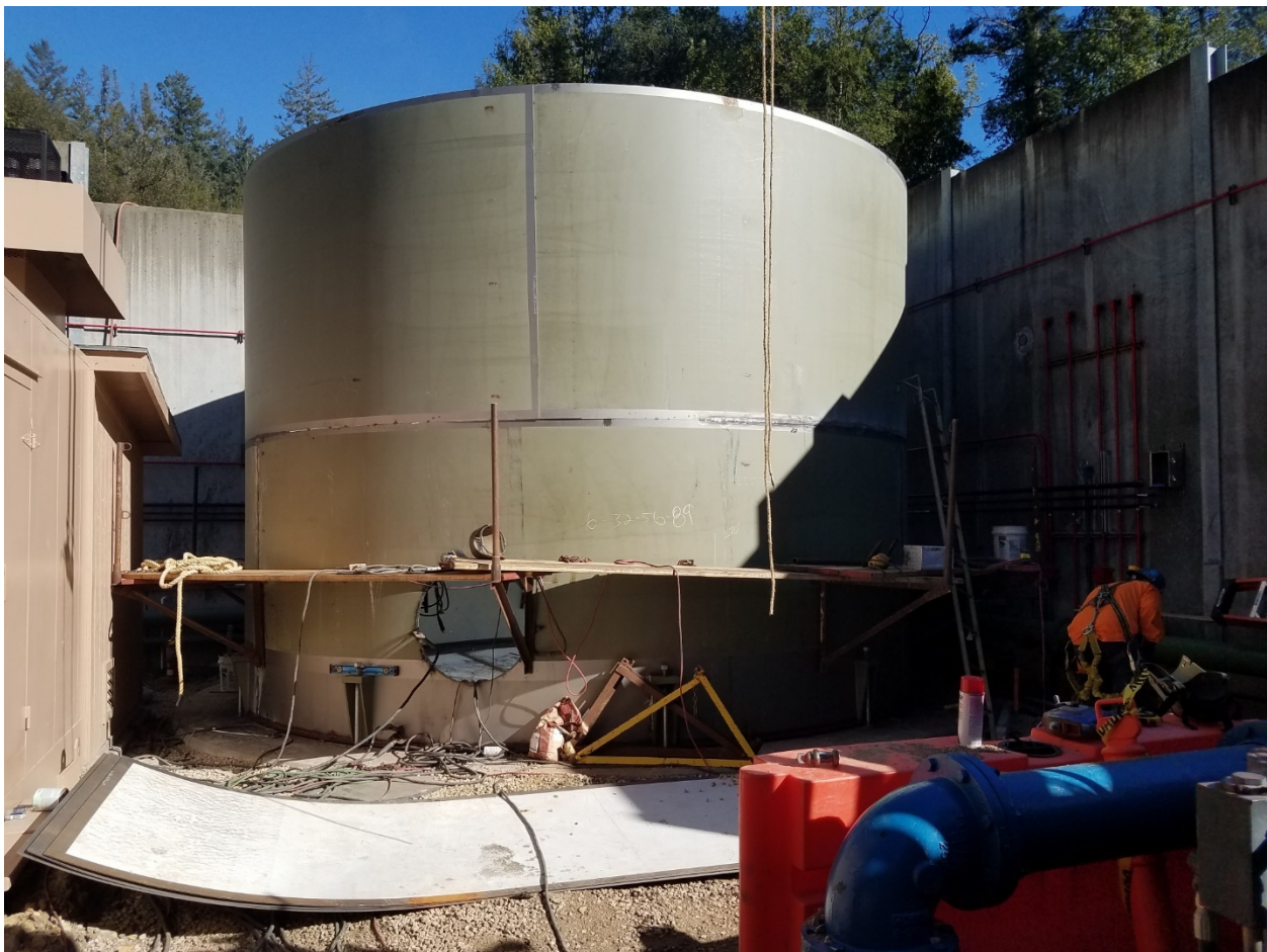
Construction of new backwash tank at Orchard Run Water Treatment Plant
