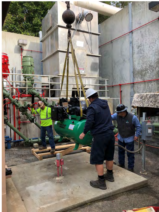
Ratepayer dollars at work – Orchard Run Water Treatment Plant
