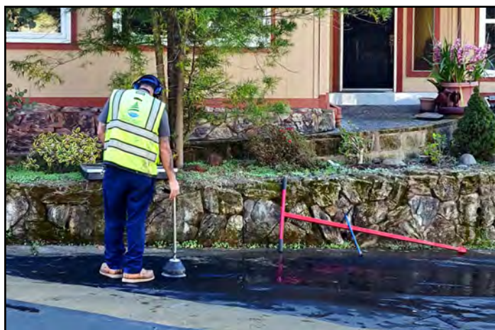
First step in finding the source of the leak is by listening with a stethoscope. Shhh! We had to turn off the fountains.
