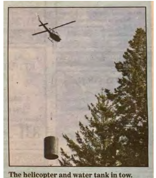
The helicopter and water tank in tow.
